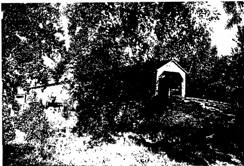
COVERED BRIDGE, CYNTHIANA
